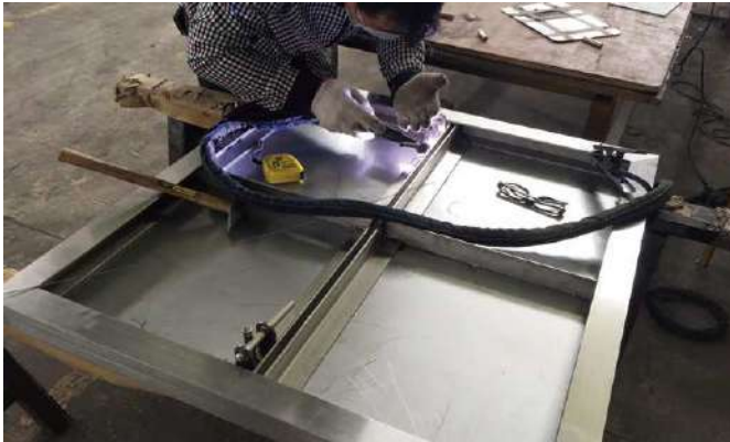
不銹鋼焊接 Stainless Steel Welding
