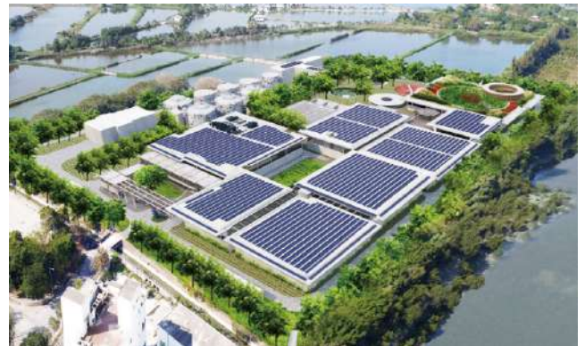
Yuen Long Water Purification Facility Phase I 元朗淨水設施第一期
